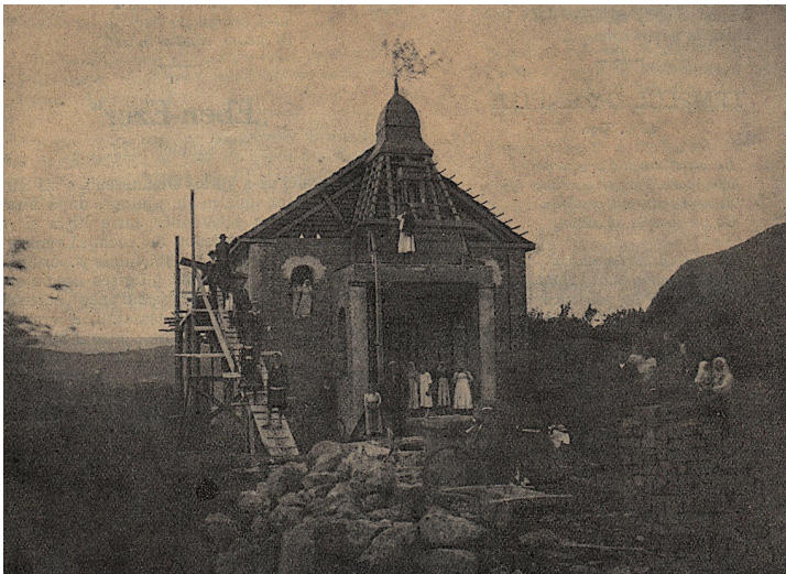
Construction of the First Baptist Church in Cluj (Source: https://bisericamanastur.ro/ )
